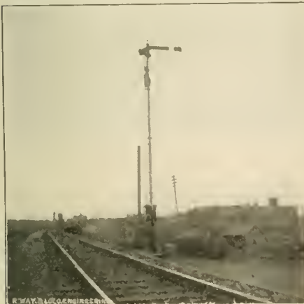
ELECTRIC SLOT INTERLOCKING SIGNAL AT ENTRANCE OF NEWARK BRIDGE OVER THE PASSAIC ON THE D. L. & W. MARKED D IN DIAGRAM.
